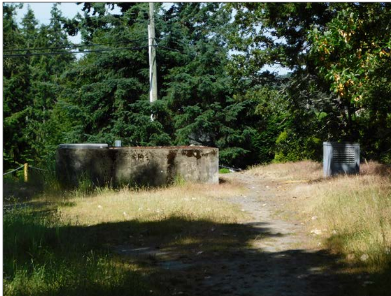
Photo 4 – Municipal water line and associated infrastructure constructed through the Site, as well as the northern portion of the Site.
