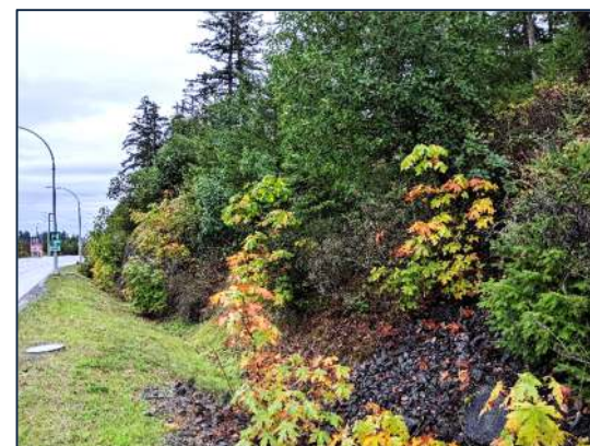
Photo 42. Northeast view of the ditch along the east side of Watkiss Way.
